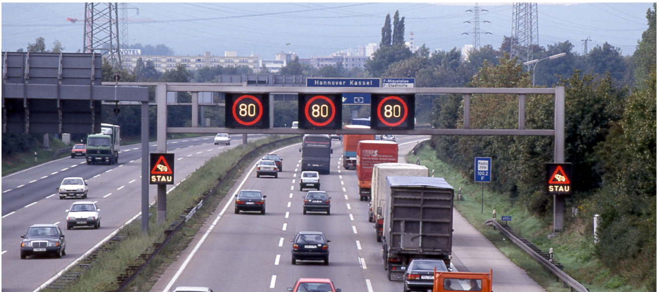
Figure 6. Managed Motorway technology in Frankfurt am Main, Germany, the VMS attached to the gantry pillars capable of displaying warnings of congestion and adverse weather conditions
