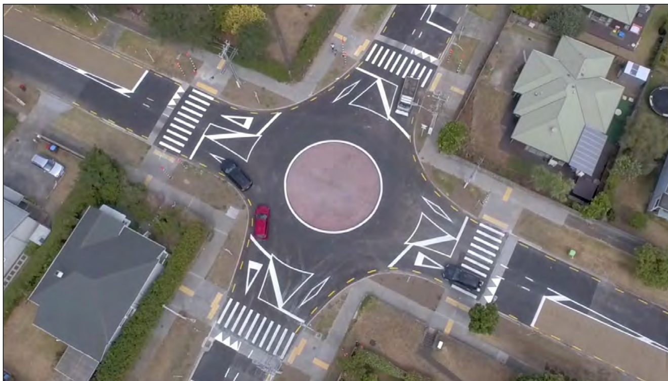
Figure 6. Drone photo of the roundabout shortly after completion
