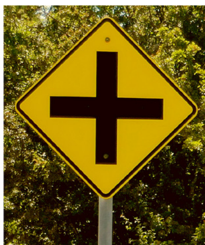
(b) Warning sign on the opposite leg (approaching Give Way)
