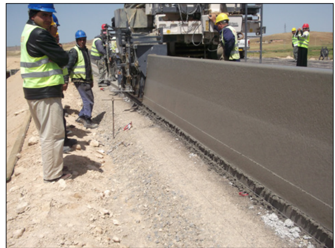
(b) Separator with 3 cm slump
