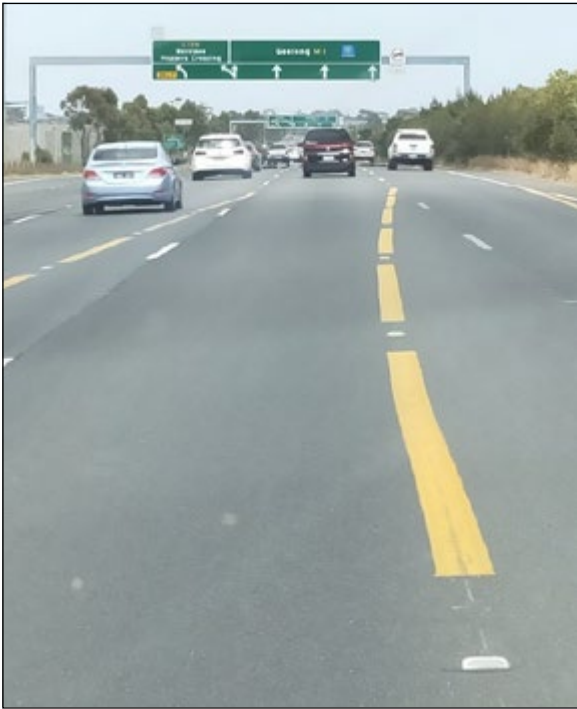
Figure 2: Example of confusing lane markings
